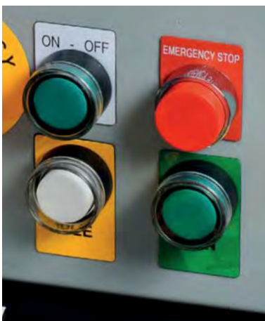
Control Panel Labels
